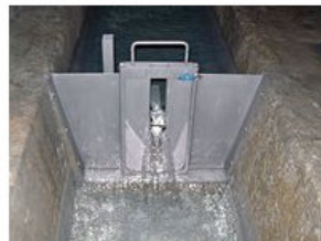
Manual Leakage Water Measurement
