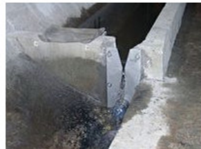
Manual Leakage Water Measurement
